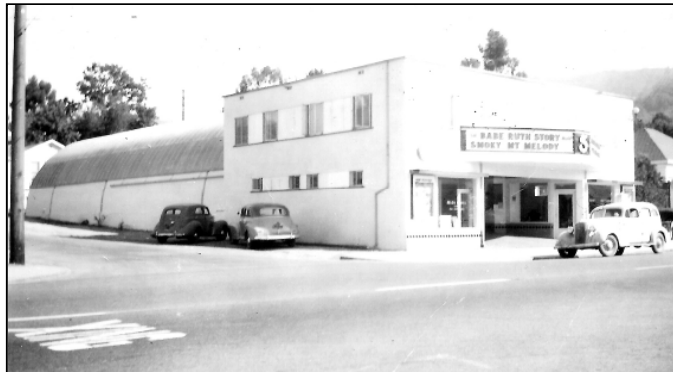
This circa 1948 photo of the Saratoga Theatre shows how a separate lobby and retail structure was added to the Quonset-built auditorium. It was demolished in the mid-1980s.
